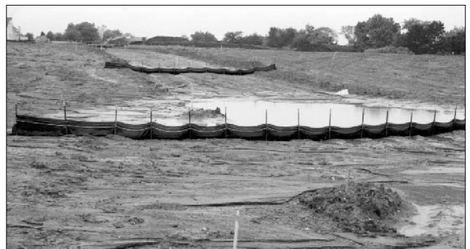
Properly installed silt fence detains water for sedimentation to occur
